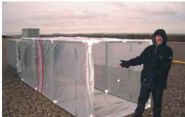
Figure 6 - Temporary ductwork on outdoor air intake allows pitot tube traverse.
